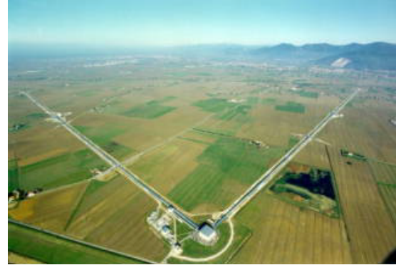
Figure 1.1 — Left: A classic Michelson interferometer consists of a laser, a 50/50 beamsplitter, two test mass mirrors and a photodetector. One can think of the gravitational wave as modulating the effective refraction index of the vacuum, thereby shortening the length of one arm while expanding the length of the other. Right: Photograph of the French-Italian VIRGO detector with an armlength of 3 km.
