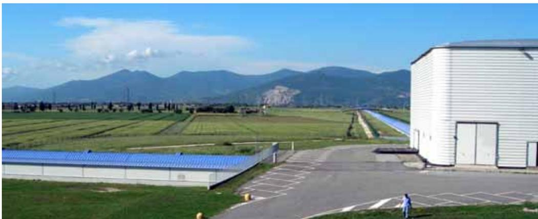
Figure 1.7: The VIRGO interferometer at Cascina, Italy. Both 3 km long arms of the detector can be seen, meeting at the central station (right hand side) which houses the input and output optics.
